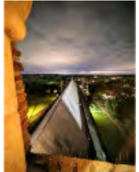
View westward from the walkway
