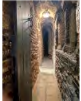
Walkway to Tower
